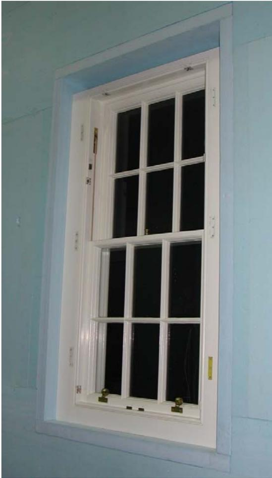
**Figure 5** Window located in central mask wall of guarded hot box
